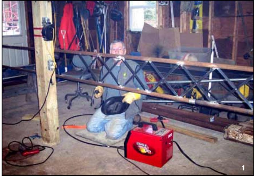
**Photo 1:** Superintendent Marc Arsenault building the Ground Line's new signal bridge . **Photo 2:** The complete signal bridge, ready to bring to the track.
